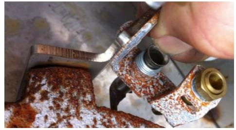
e. After removing the pilot orifice, clean thoroughly with soapy water and a soft bristled brush (toothbrush).
